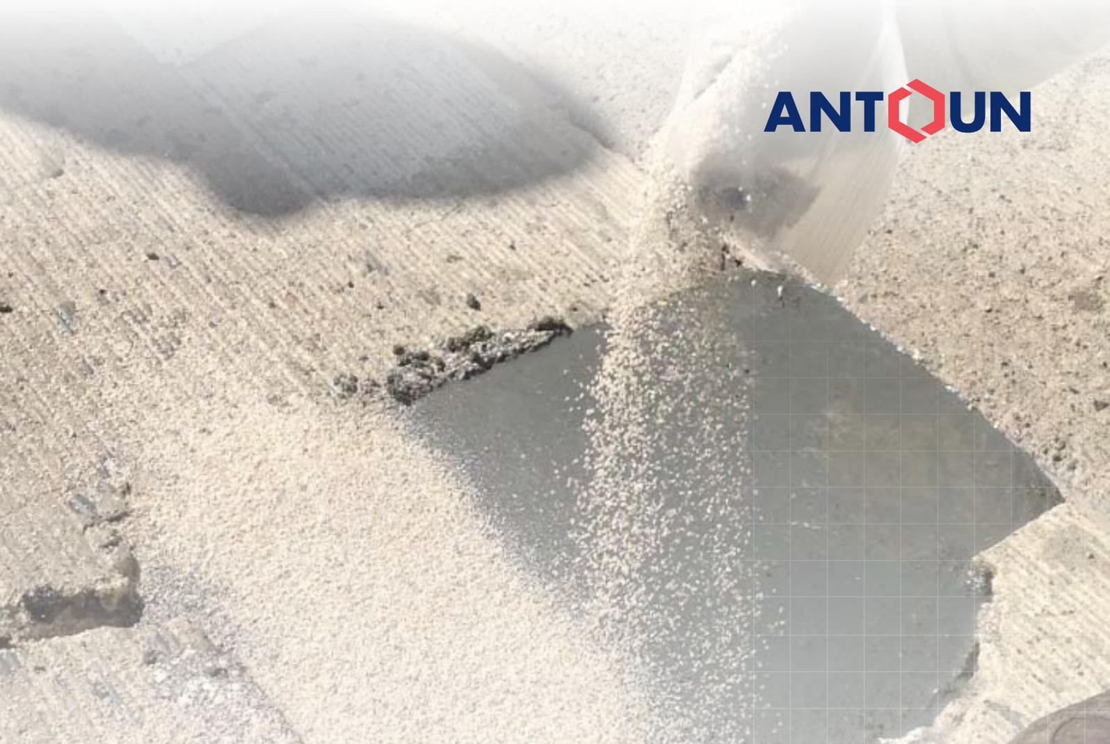
A close-up photograph showing a person's hand in a white glove pouring a grey, granular repair material into a hole in a concrete surface. The material is being applied to a prepared area, and the surrounding concrete is light-colored and textured.
